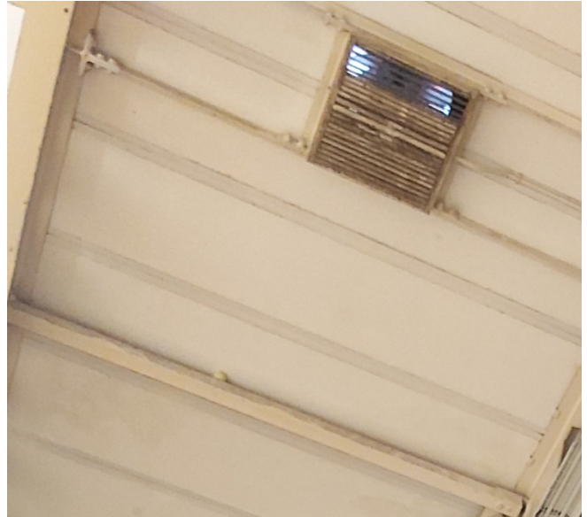
Sport Hall Stramit board cassette with liner (Viewed from below)
